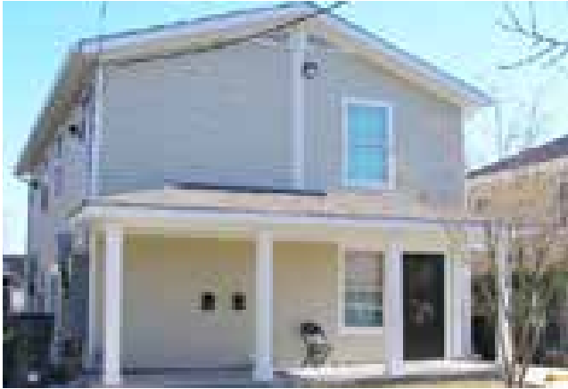
1112 N Rocheblave after rehabilitation by HANO
