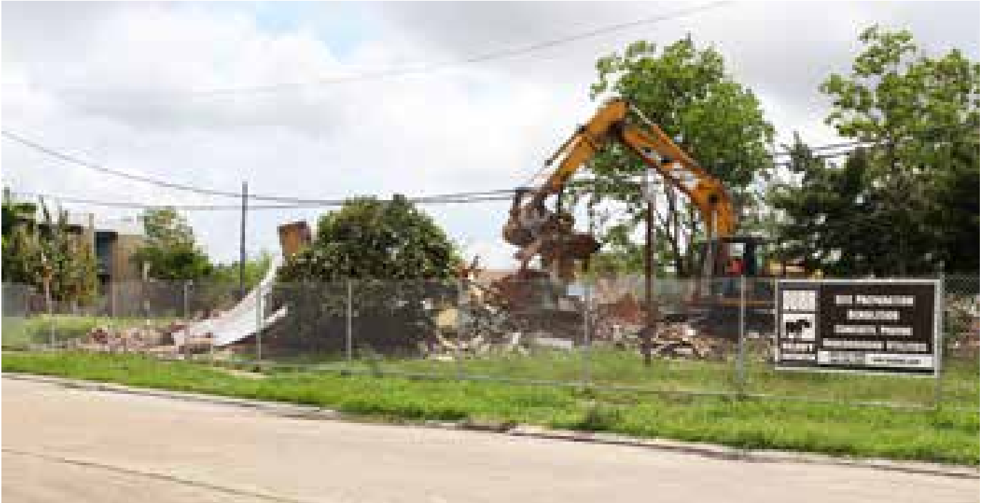
Christopher Park Demolition
